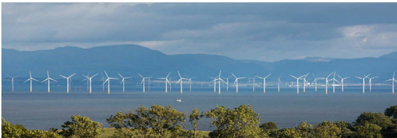
Robin Rigg Wind Farm
